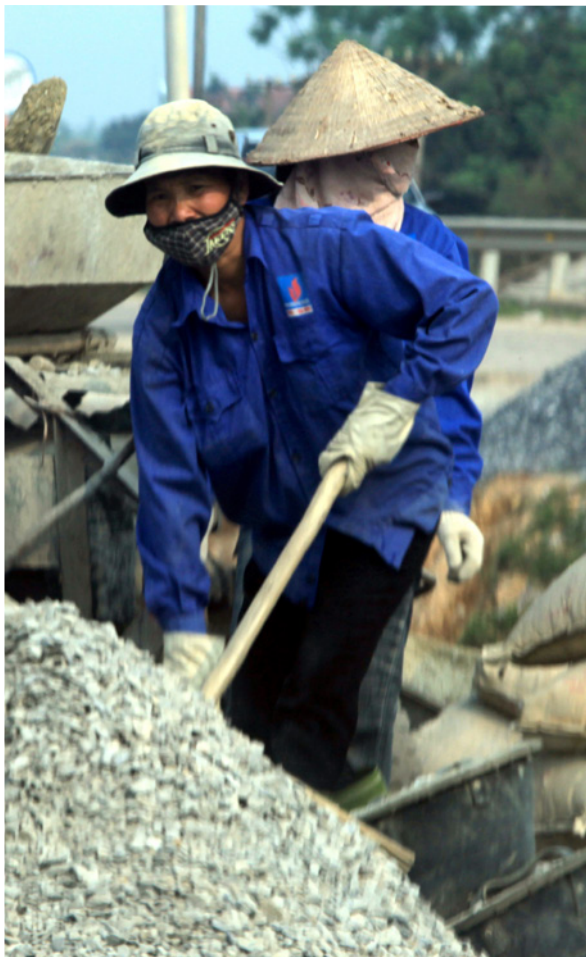
Construction workers at work. © ILO/T. Van Vi
